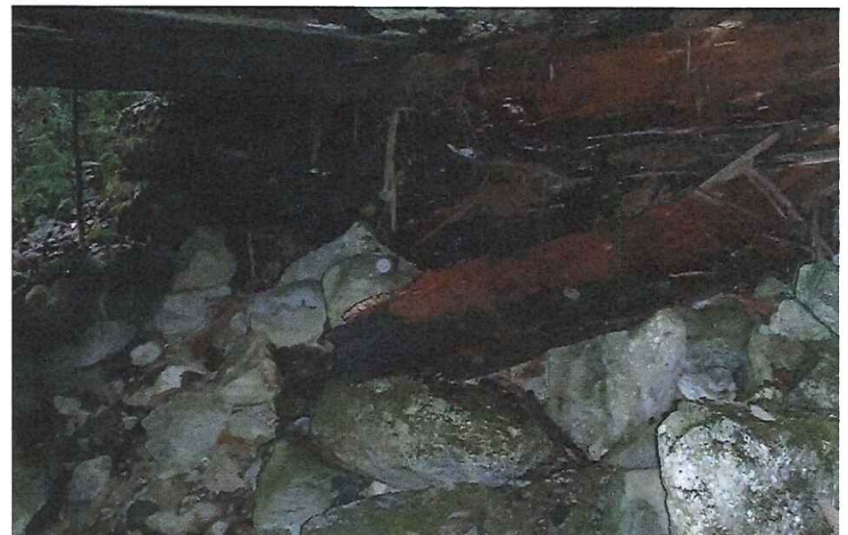
CK2255 Right Abutment
