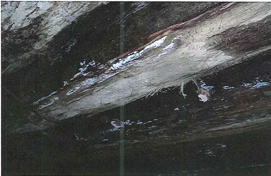
CK2255 Conc on Stringers
